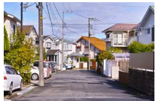
Via Power Lines (from one building to another)
